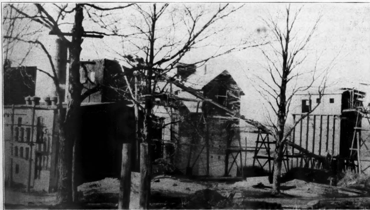
Screening Plant at Right with Sand Conveyor to Brick Plant at Left
